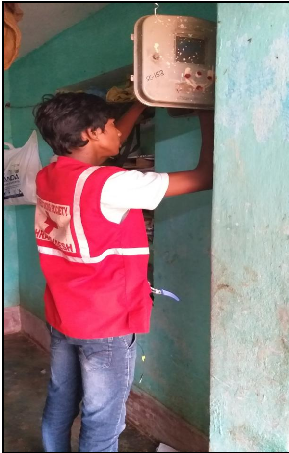
Repairing Electrical wiring
