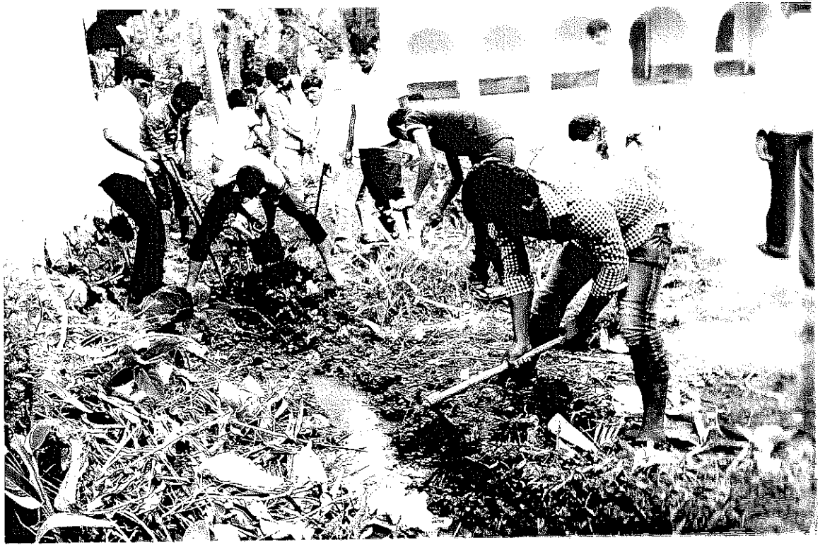
our volunteers digging a katcha drain
