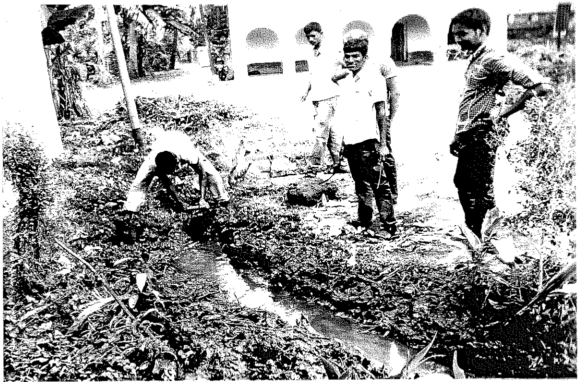
our volunteers digging a katcha drain
